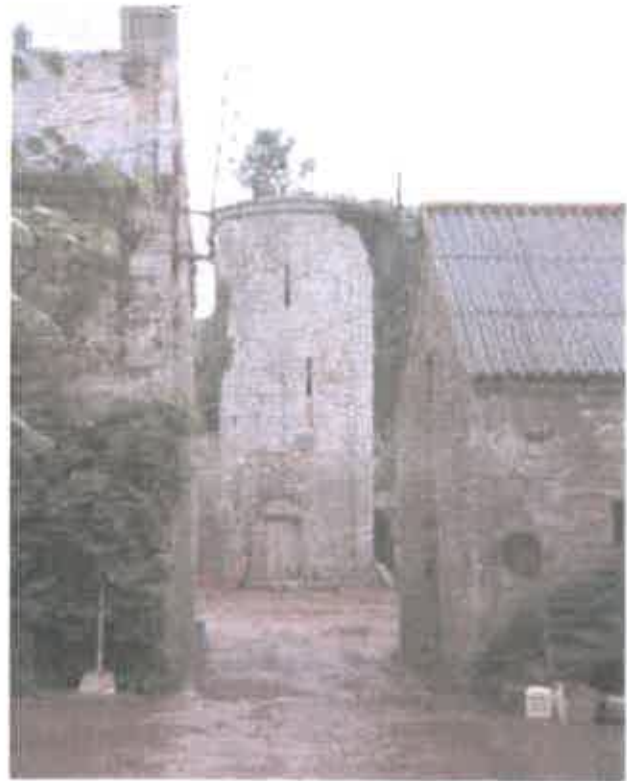
Figure 3. The Saint-Aloüarn Manor in Geungat, September 1998.
