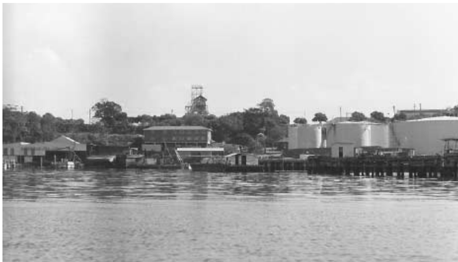
View of Woodleys Boatyard and BP Refinery from the Harbour
